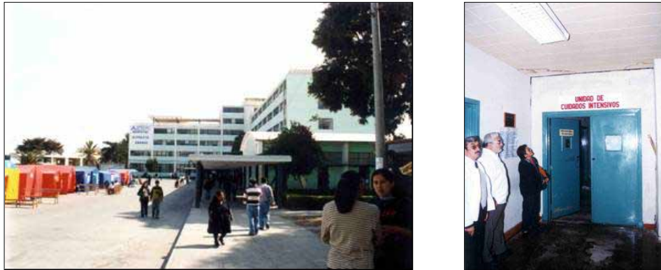
Fig. 5. “Hipólito Unanue” hospital in Tacna had damage to non-structural walls and sanitary installations.
