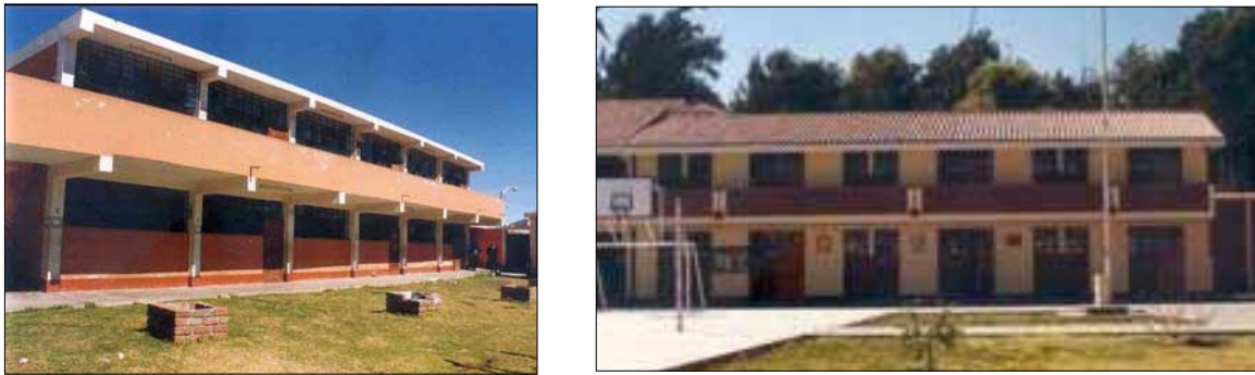
Fig. 4. Traditional school without damage due to infill wall at rear facade (left), and new school buildings featuring strong columns in the longitudinal direction without any damage (right).
