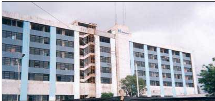
Fig. 12. Main building of the Arequipa hospital, during the construction retrofitting process.
