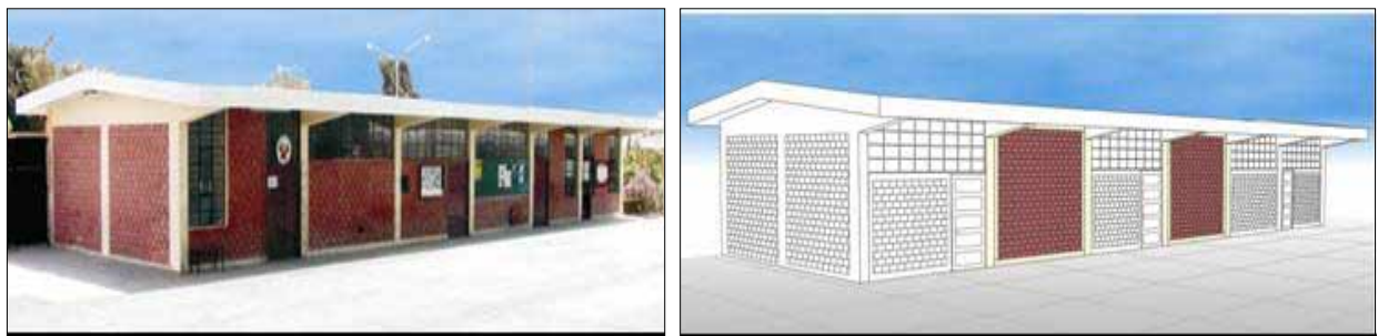
Fig. 8. One story school building damaged after the 2001 earthquake (left) and projected retrofitting in the longitudinal direction (right).
