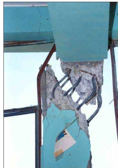
Fig. 2. “Angela Barrios” school in Moquegua: interior column general failure (left), and exterior column failure (right).
