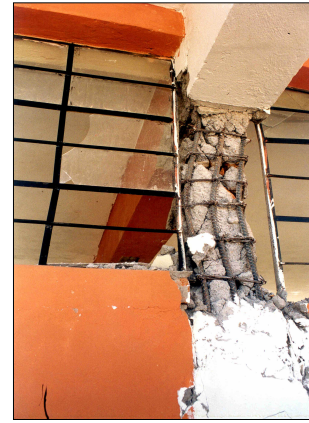
Fig. 1. “Casimiro Cuadros” school in Arequipa: old and new blocks (left) and short column failure in old block (right).
