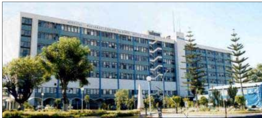
Fig. 10. Main building of the Arequipa hospital before the retrofitting.
