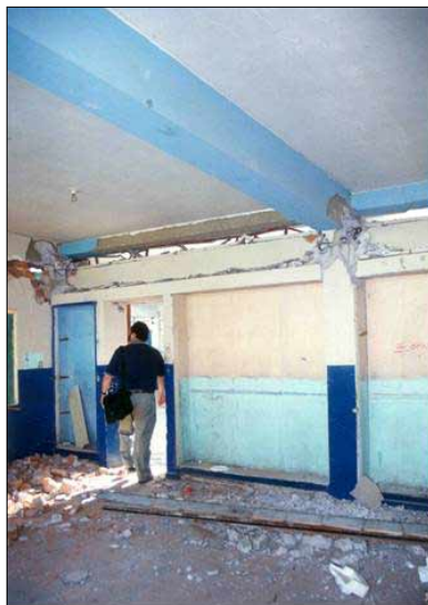
Fig. 2. “Angela Barrios” school in Moquegua: interior column general failure (left), and exterior column failure (right).
