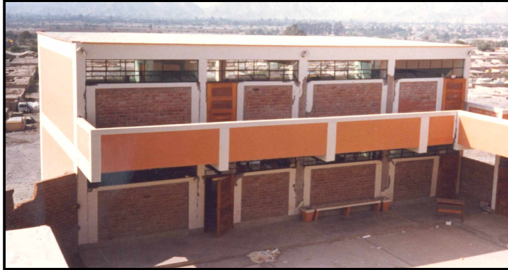
Figure 1. Typical Peruvian school building
