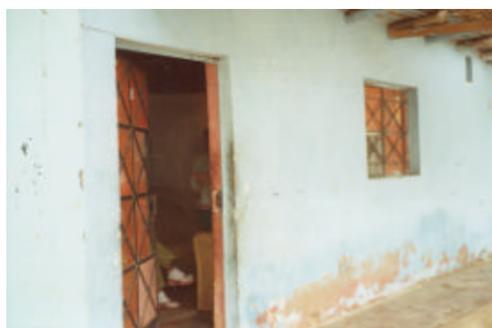
Figure 16. Partly retrofitted house in Ica Central had no damage
