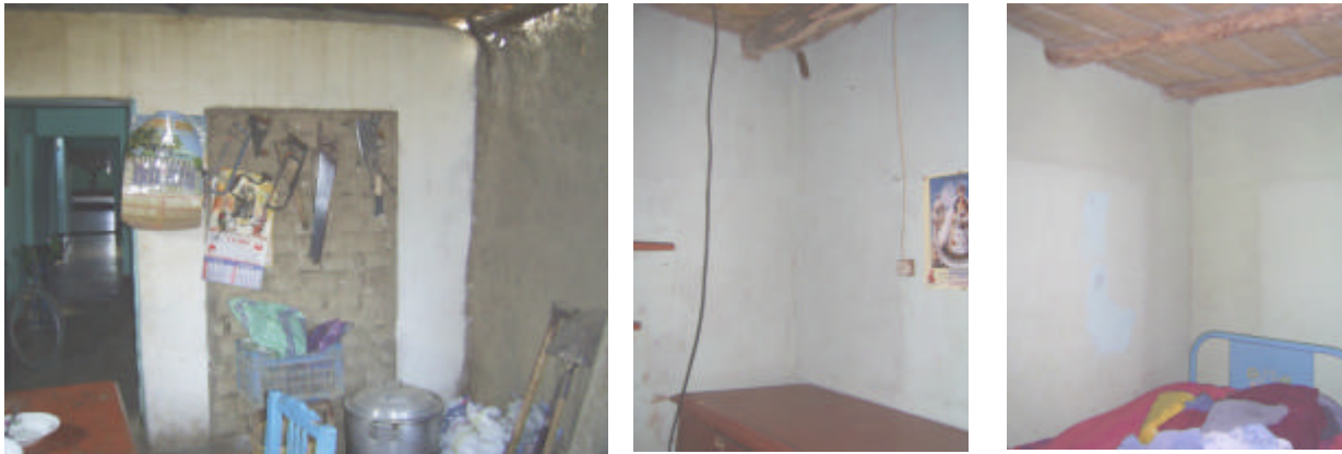
Figure 10. Pachacutec retrofitted adobe house without damage
