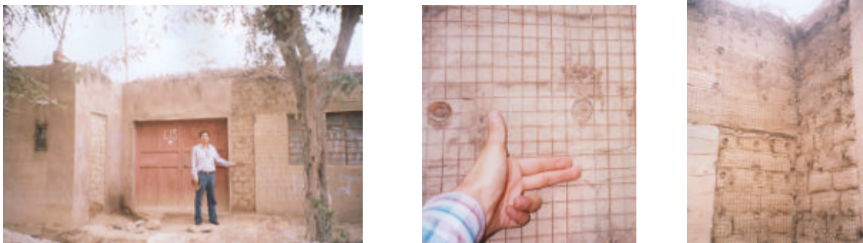
Figure 12. Partly retrofitted Parcona house without damage
