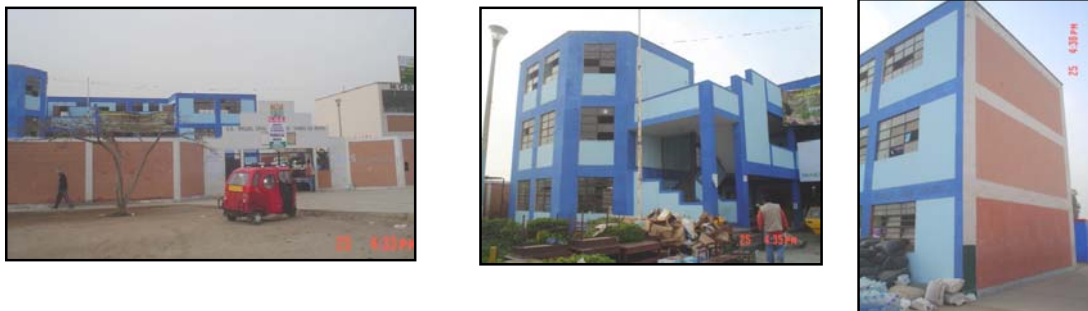
Figure 5. School in Tambo de Mora, Chincha had slight damage.
