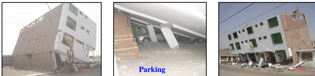
Figure 9. Soft story and torsion.
