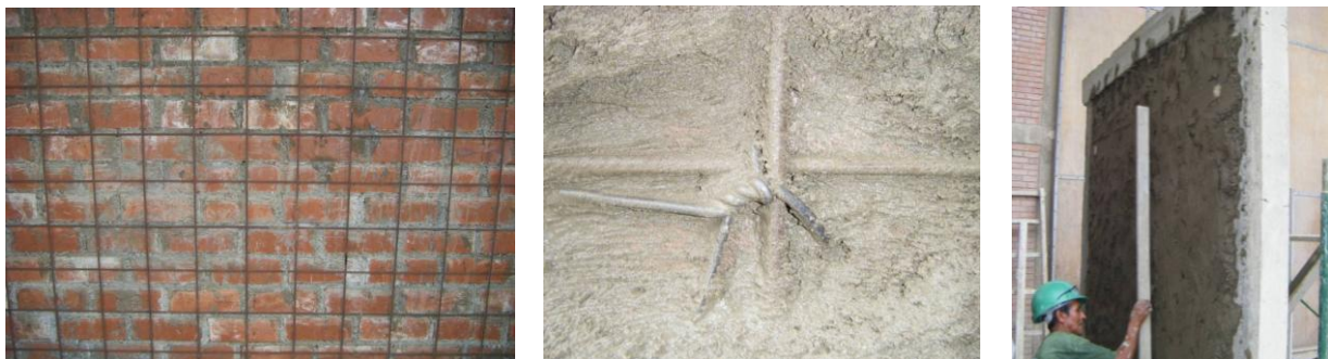
Figure 5. Wall W2: wire mesh (left), connector (centre), and final cover (right).
