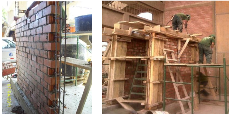
Figure 4. Construction of masonry walls W1 and W2.
