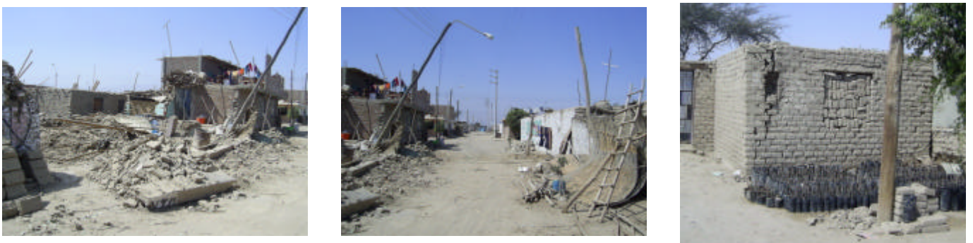
Figure 11. Traditional adobe houses with damage in Pachacutec
