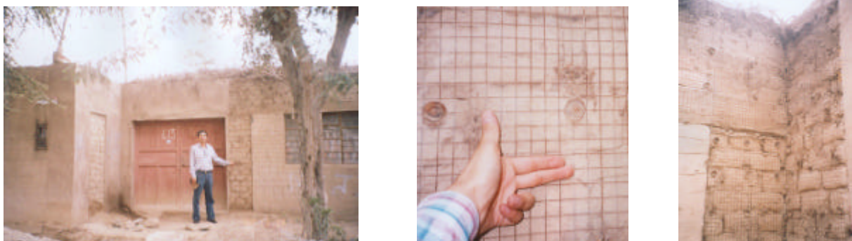
Figure 12. Partly retrofitted Parcona house without damage
