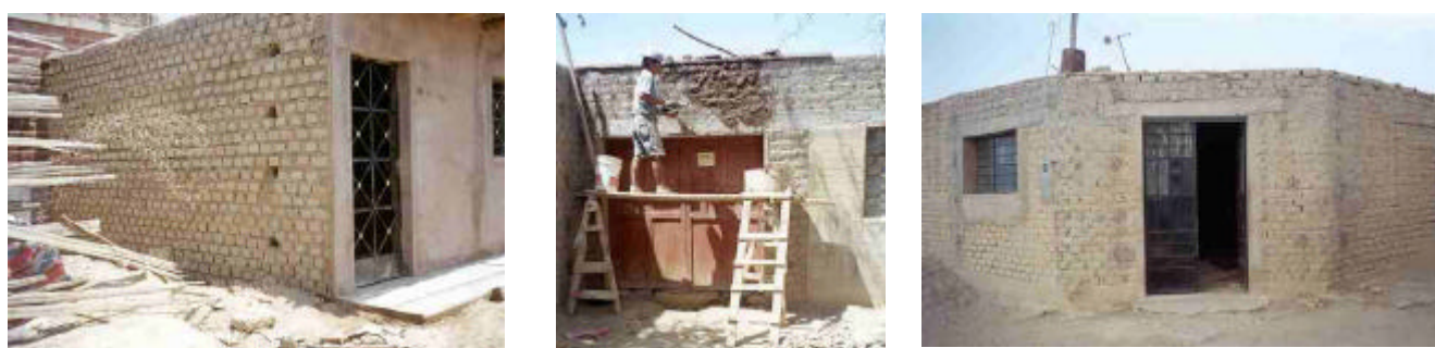
Figure 6. Demonstration adobe houses in (left to right) Ica Central, Parcona and La Tinguña, during reinforcement in 1998.
