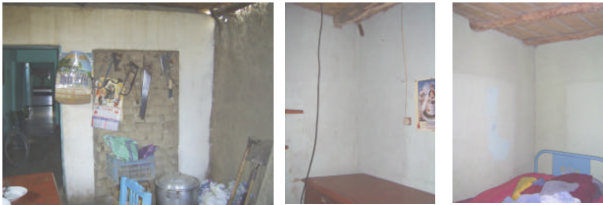
Figure 10. Pachacutec retrofitted adobe house without damage
