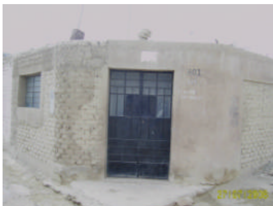
Figure 14. Partly retrofitted house in La Tinguiña had no damage.
