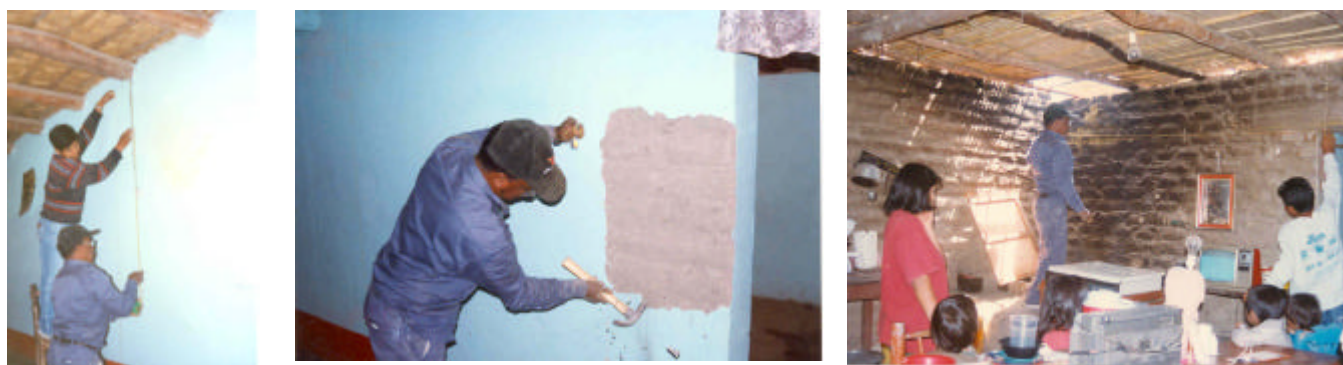
Figure 5. Adobe house in Pachacutec retrofitted in 1998 (left to right): marking vertical strip, removing existing covering, and marking horizontal strip.
