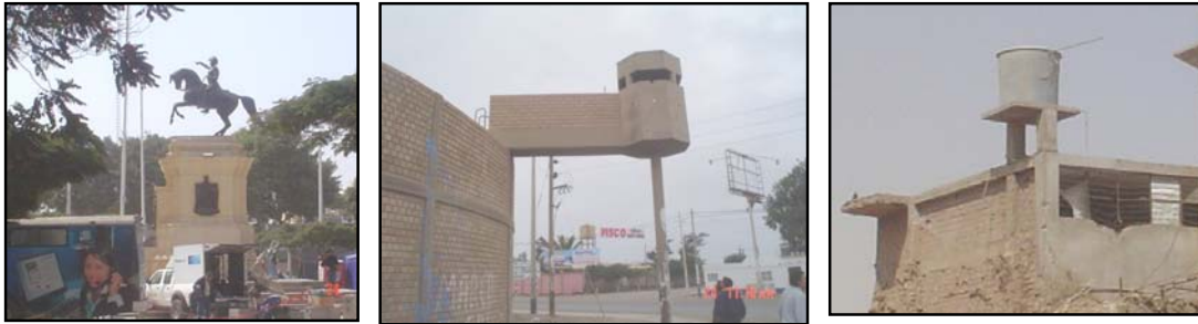
Figure 3. Evidences that the Pisco earthquake can be qualified as moderate.
