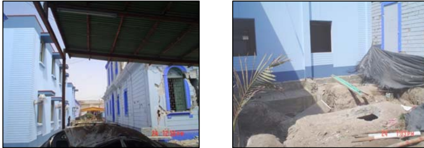
Figure 6. Pisco hospital with rigid foundation in new block (right)
