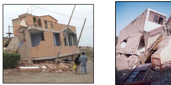
Figure 10. Low wall density
