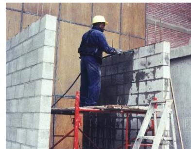
**Figure 9: Treatment by watering of walls W4 and W5**
