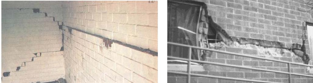
**Figure 1: Sliding failure in masonry walls, Chile (1985) and Northridge (1994)**
