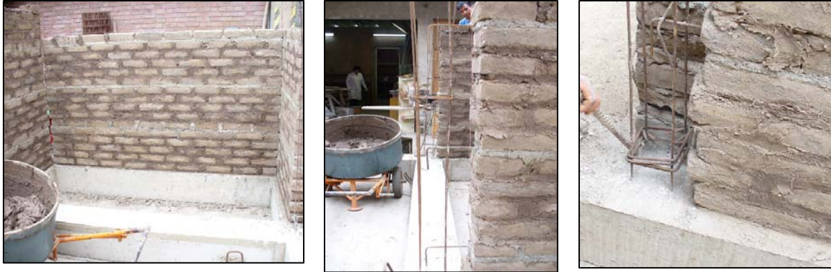
Figure 5: Details of the first story construction
