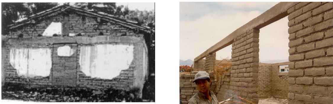
Figure 2: Good behavior of one-story adobe houses confined by RC elements, Ometepec Mexico [4] (left) and Nasca Peru [5] (right)
