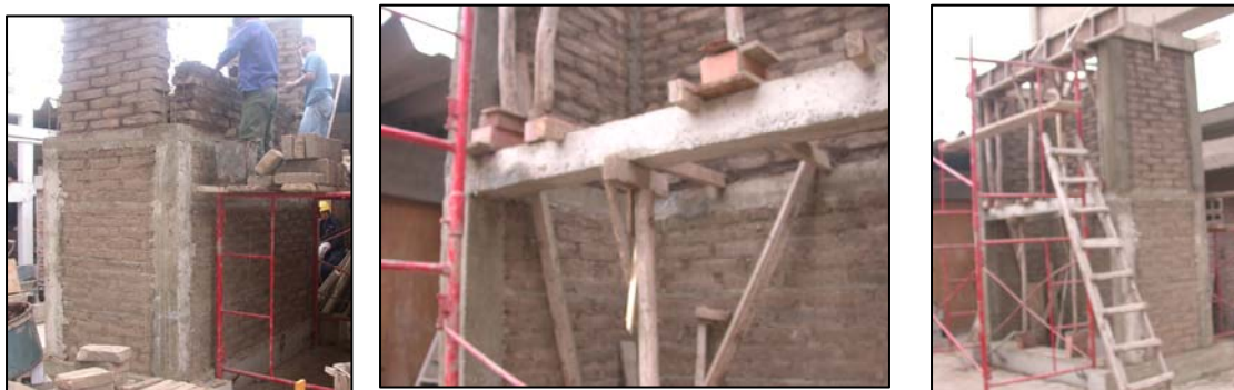
Figure 6: Details of the second story construction
